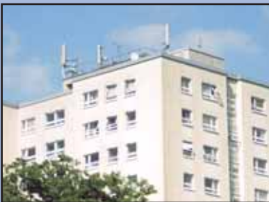
Typical rooftop telecommunications equipment
